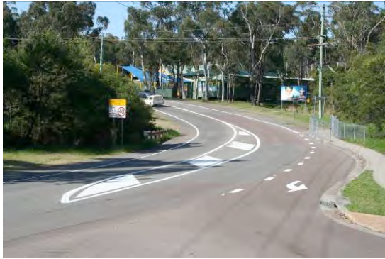
Photograph 3 Fenced footpath across culvert between the railway station access and the college.
